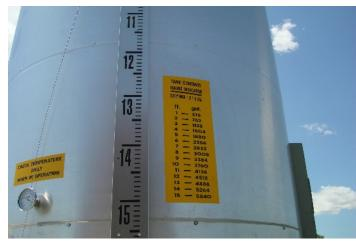
Emulsion quantity measuring system consisting of stainless steel float, cables and indicator board.
