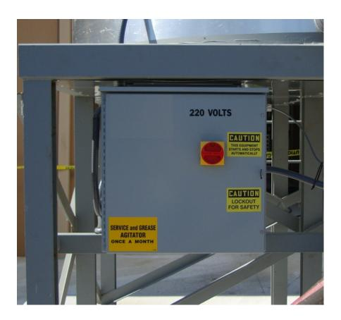
Electrical components in a single lockable weather proof NEMA 3R enclosure
