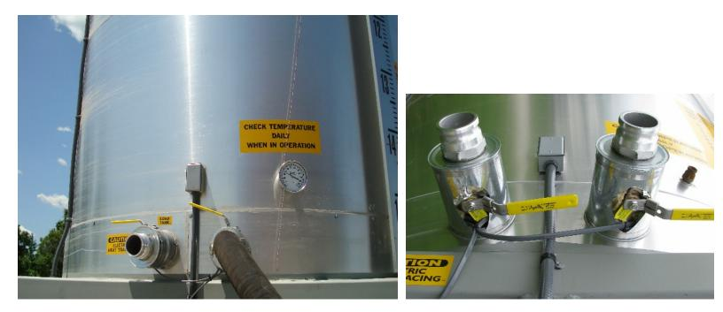
3" Ball valves heated with 220v heat tape. Insulated an wrapped.
