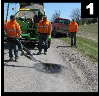
Apply Tack Coat
