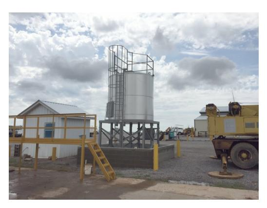
Complete Safety cage system on access ladder and top of tank. With anti-fall bars in access hatch.
